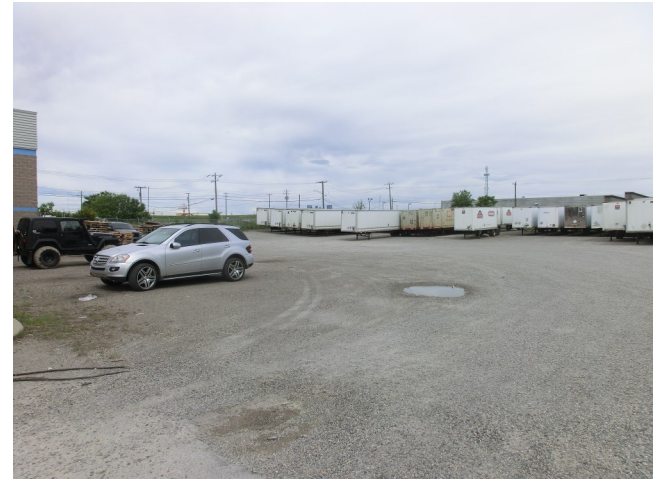
REAR YARD, GRAVELED/COMPACTED 1.56 ACRES
