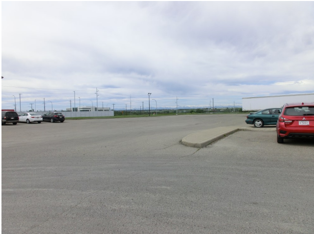
FRONT PAVED PARKING/YARD 1.08 ACRES
